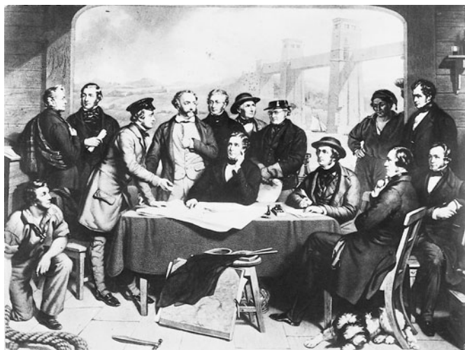
6. British engineers of the railway age, a posed group by John Lucas, ostensibly set in autumn 1849 in a hut on the edge of the Menai Straits during the hoisting into position of the tubular wrought-iron spans of Robert Stephenson's Menai Bridge (in background) on the Crewe-Holyhead railway. Stephenson is seated centre, and Isambard Kingdom Brunel on the far right. Joseph Locke (seated second from right) completed the triumvirate of great railway engineers. All three died in their mid-fifties, worn out by overwork, in 1859–60
